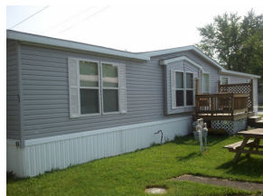
Pictured, is one of the 17 mobile homes repaired in FY 2010.
