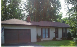
Five low-mod elderly households received home repair in CDBG FY 2010.
