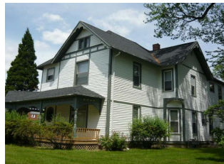
Using CDBG funds, this multi-unit housing site was made more decent and affordable in FY 2010.
